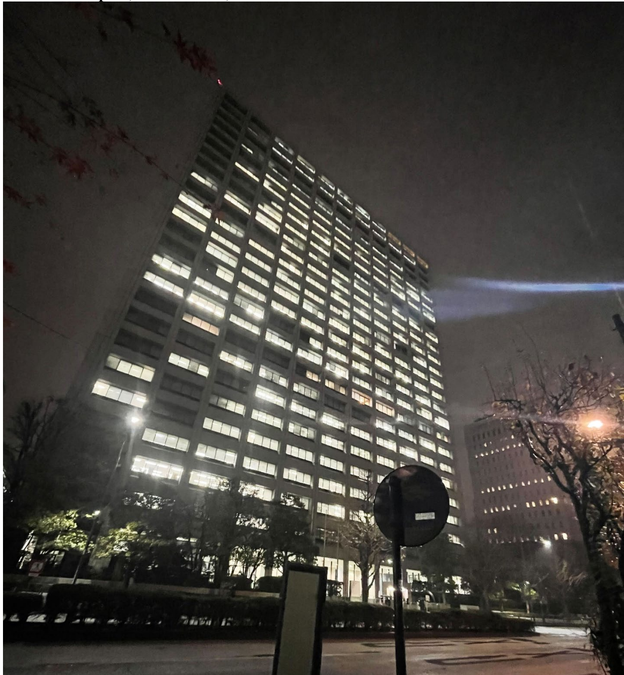
Figure S1. Central Government Building No. 5, housing the Ministry of Health, Labour and Welfare. 7:00 p.m., December 24, 2025
